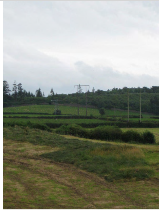
Plate 67: BK38, 39 and angle mast 40 WL45 with Jenkinstown Demesne wall in background looking SE.
