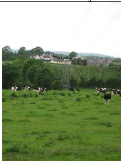
Plate 24: BK89 angle mast (WL72) looking NW.
