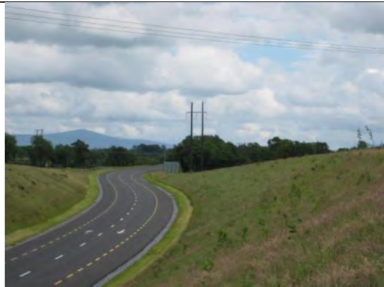
Plate 6: BK101 at edge of motorway link looking E.
