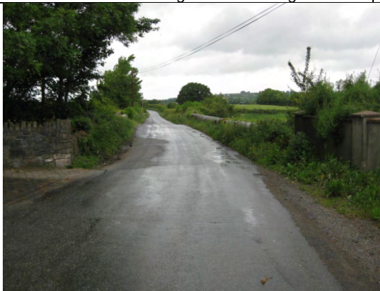
Plate 57: Protected Structure D36 Dinins Bridge Mohill looking N.
