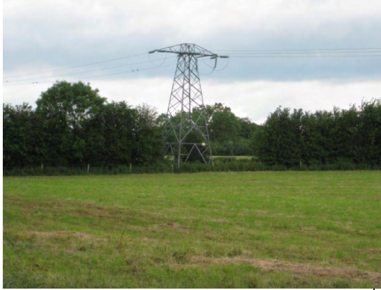
Plate 31: BK 79 angle mast WL67/68 looking N.
