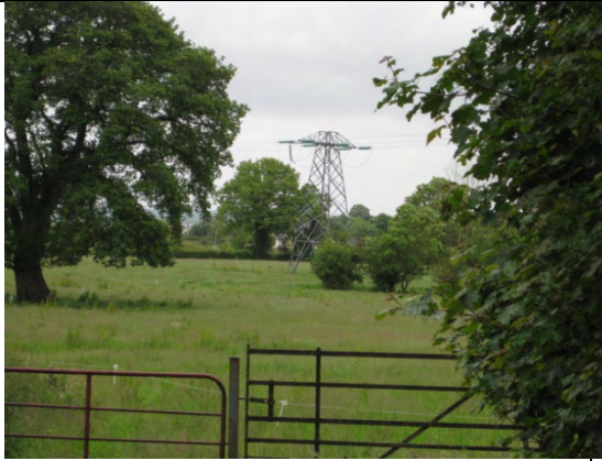
Plate 55: BK51 angle mast looking N.
