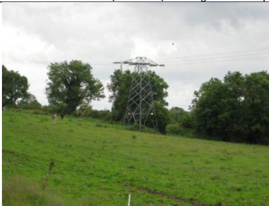
Plate 21: BK89 angle mast (WL72) looking SSW.
