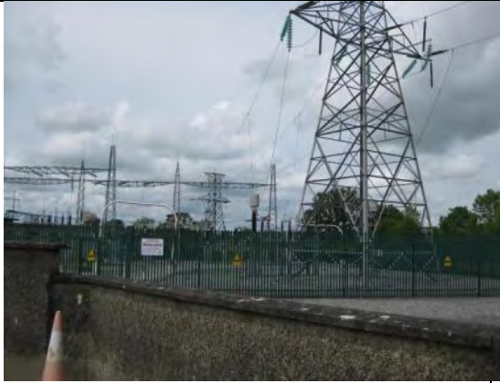
Plate 1: Existing substation at Kilkenny.
