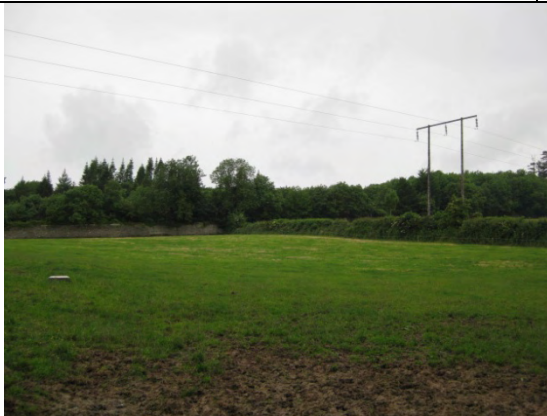
Plate 65: BK42 WL45 and Jenkinstown Demesne wall in background looking W.
