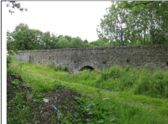
Plate 25: Roadbridge at Cellarstown between BK89 and BK88 looking N from WL 72.
