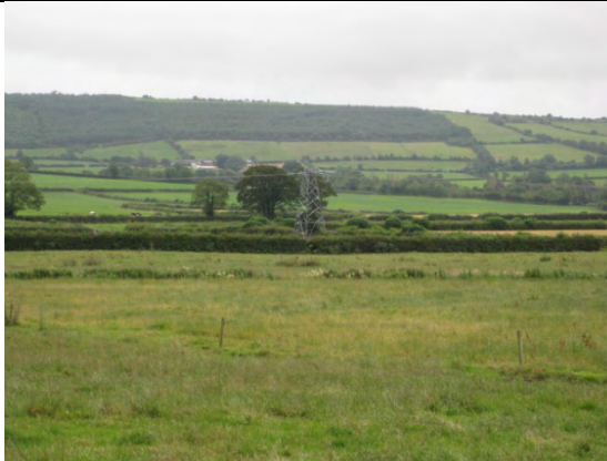
Plate 81: BK11 angle mast WL27/26 looking ESE.
